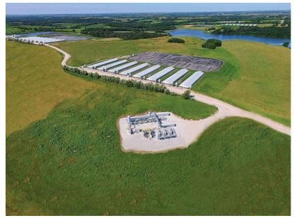
Covered lagoons allow methane gas to be captured, scrubbed, and injected as renewable natural gas into the nation's pipeline system.
